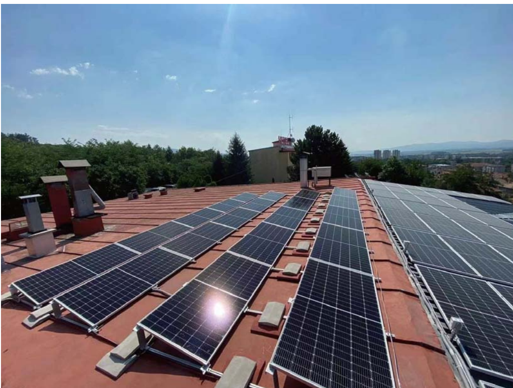
Ballasted Mounting-Bulgaria
