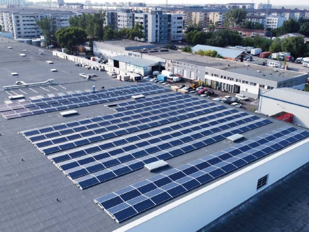
East & West Ballasted PRO-Romania
